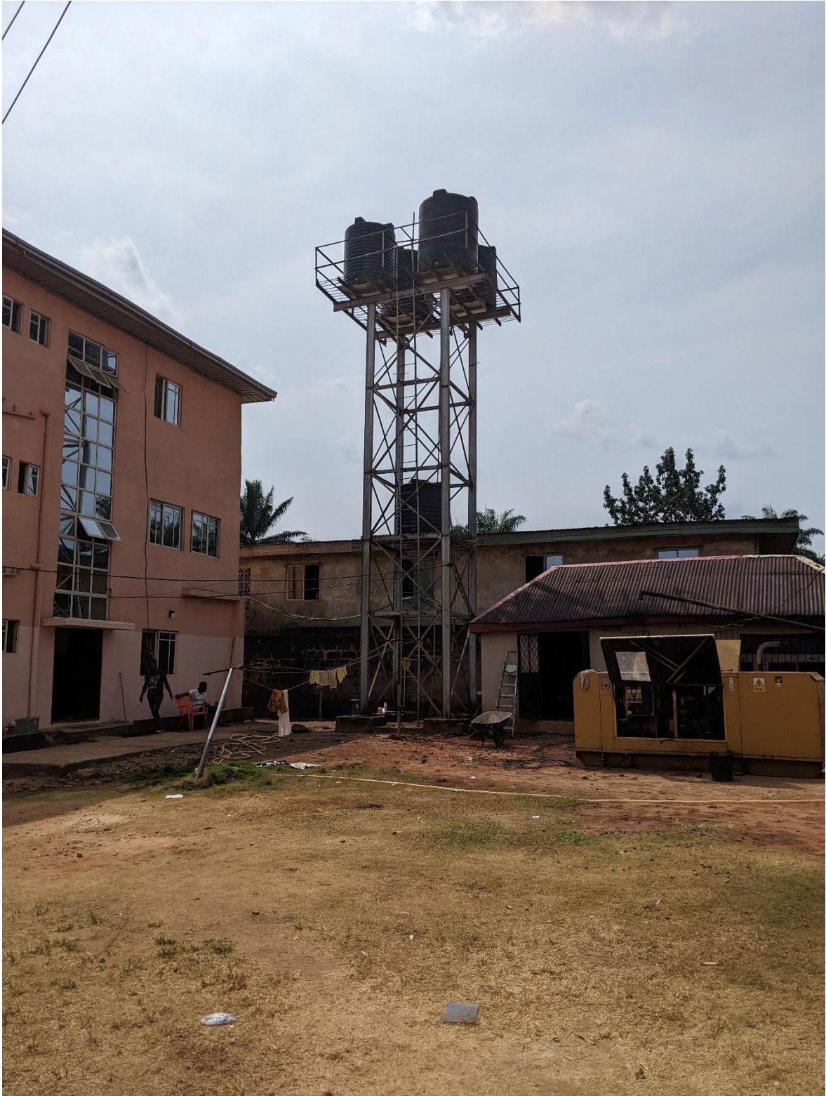
Figure 12 Water storage tower
