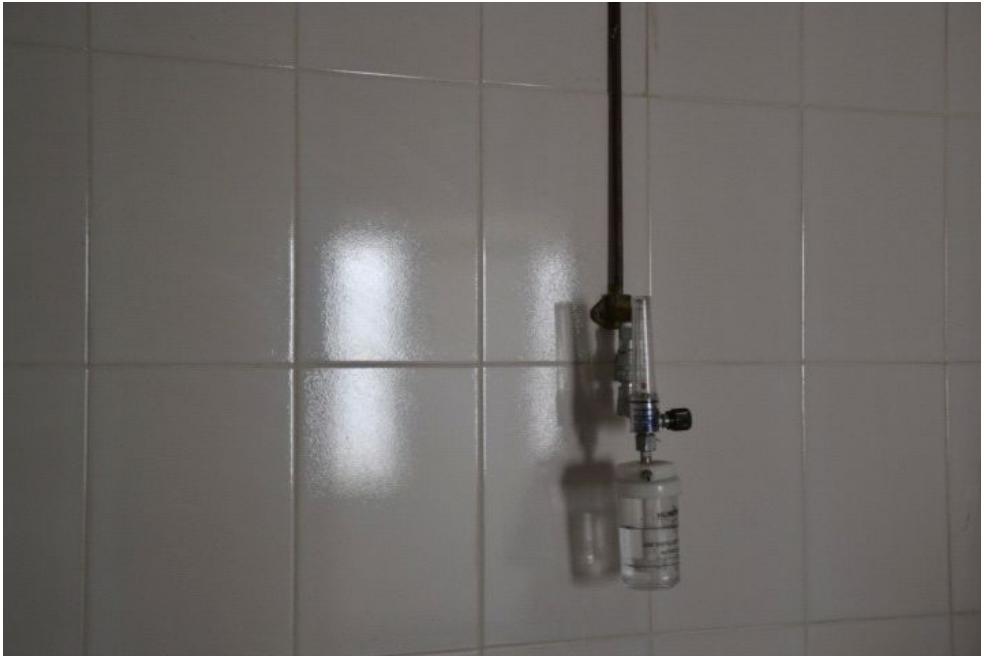
Figure 27: Sample 15: oxygen-humidifier, pow and operating theatre, ground floor and first floor – Photographer: Angelika Schirnhofner
