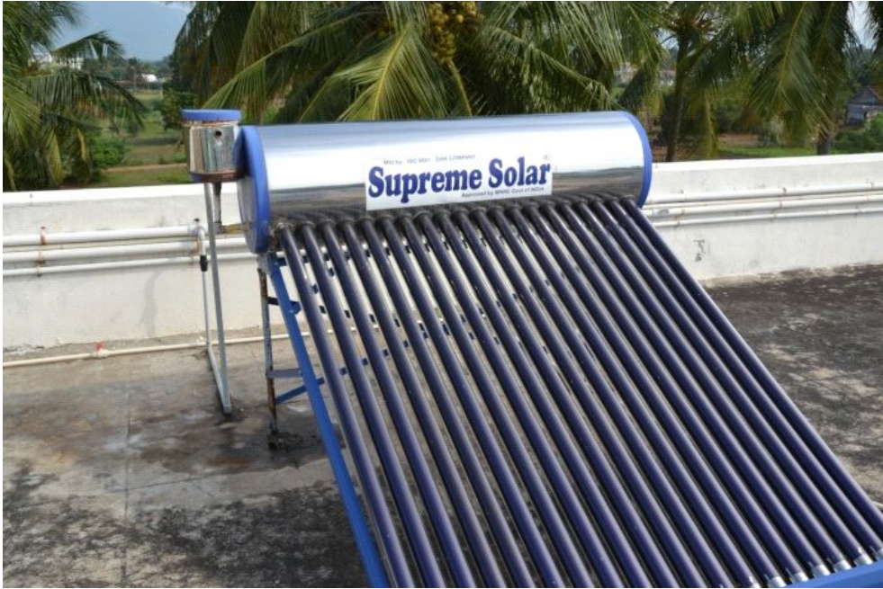
Figure17: Sample 5: solar heater – Photographer: Angelika Schirnhofner
