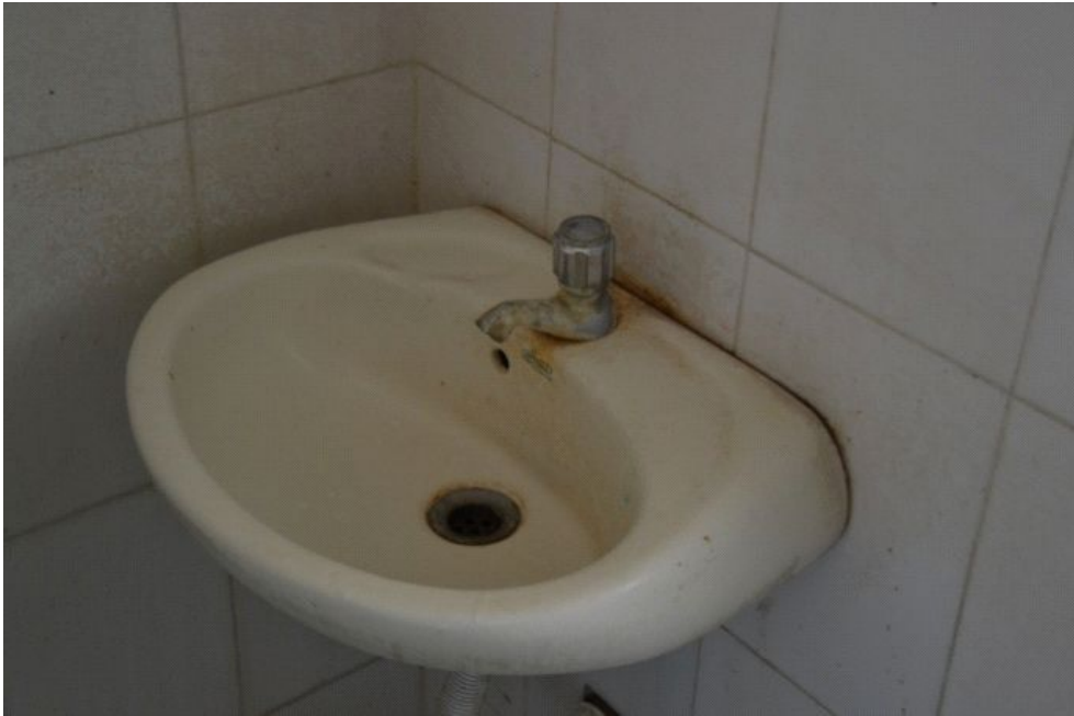
Figure 23: Sample 11: water tap room C, ground floor – Photographer: Angelika Schirnhofner
